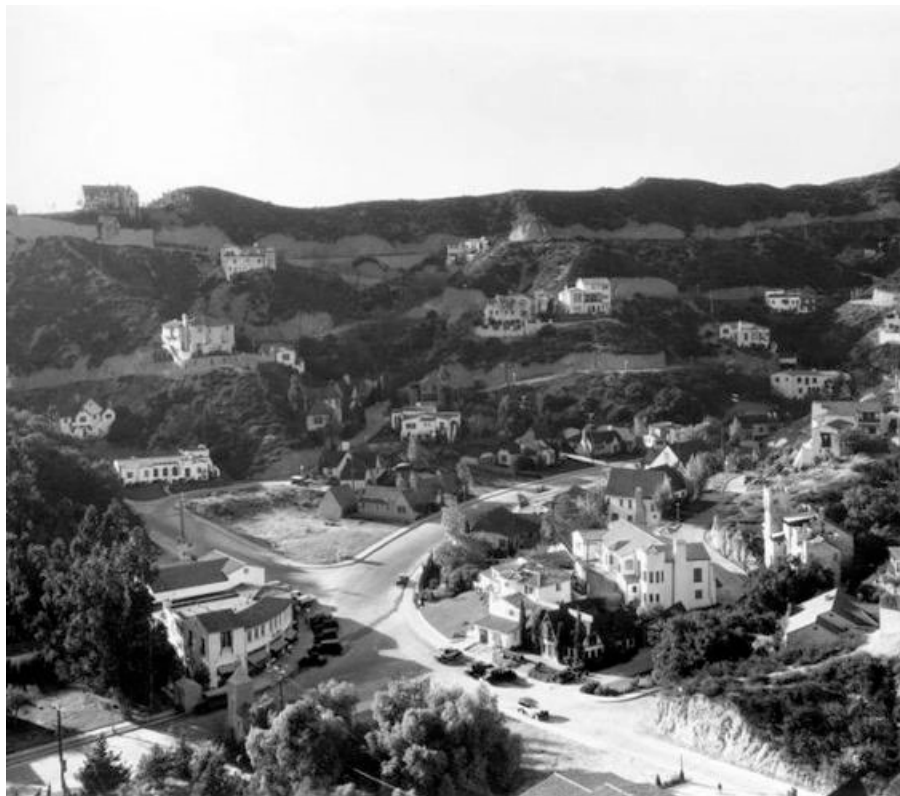
Photo 2: Development around 1928. Note the steep road cuts.
