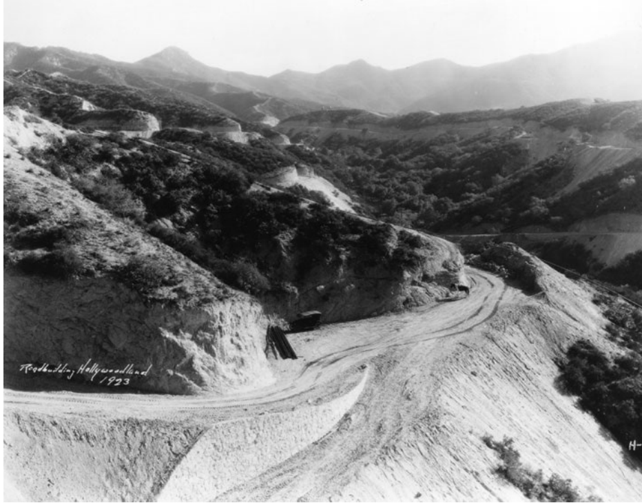
Photo 1: Steep slopes for road construction, 1923
