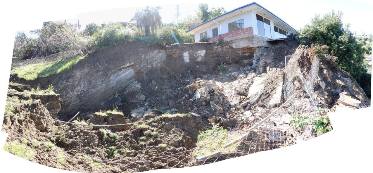
Photo 6: Landslide involving layered sedimentary bedrock, 2024
