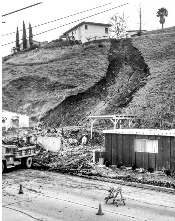
Photo 4: Soil slip/mudflow
