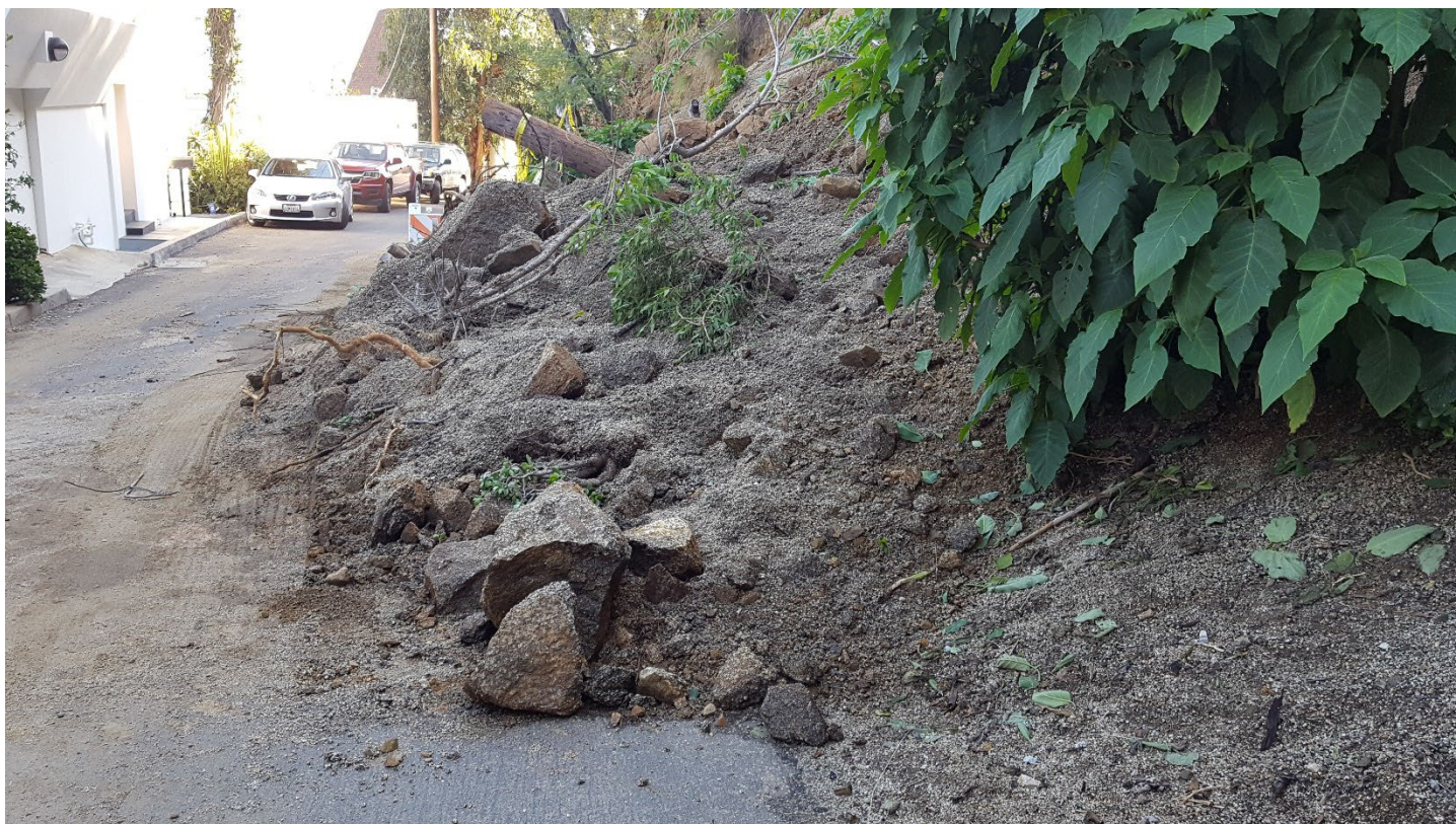
Photo 5: Rockfall from granitic rock
