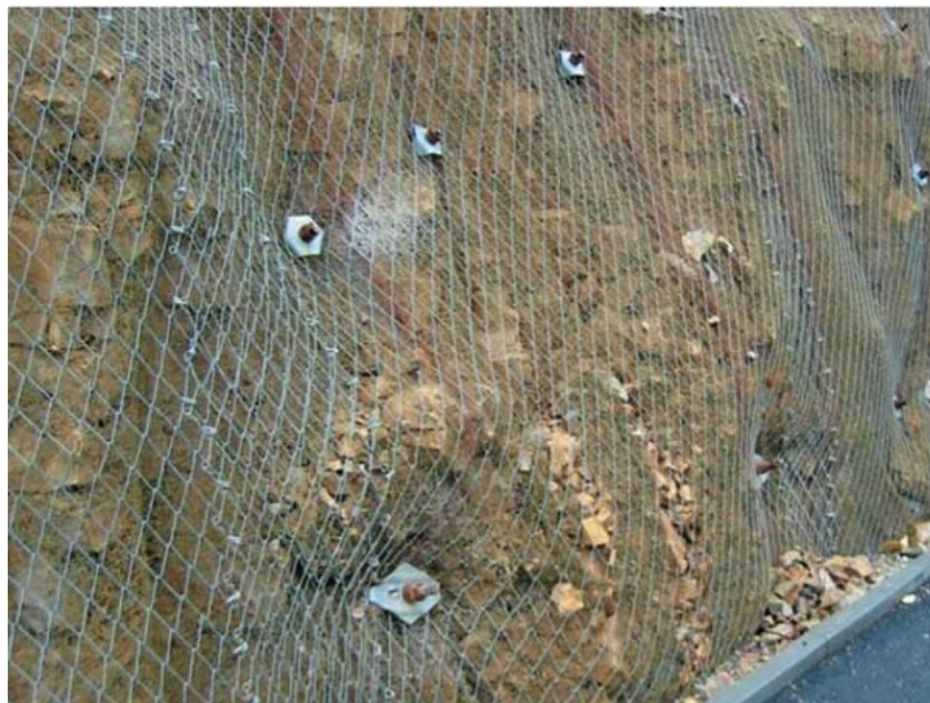
Photo 10: An unstable rock slope repaired with anchored steel mesh.
